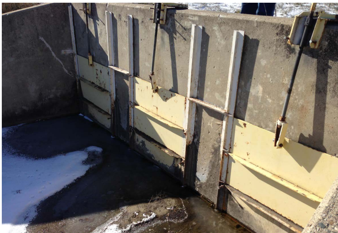
Figure 2-3. Okabena Creek bypass flood gates at Oxford Street.
