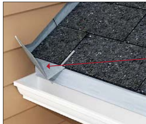
Kickout flashing
