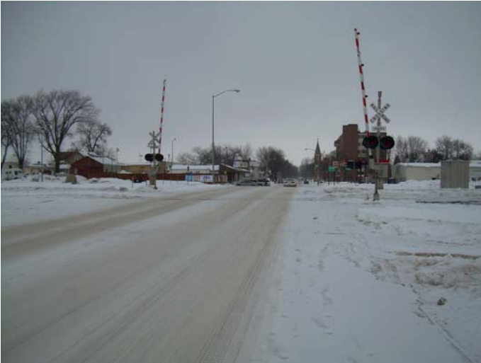
Looking Northwest– Southeast of Crossing
