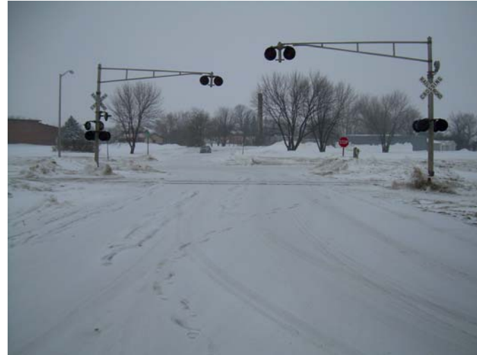
Looking Northwest, Southeast of the Crossing
