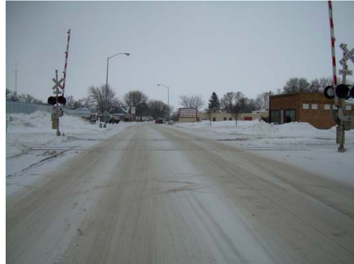
Looking Southeast, Northwest of the Crossing
