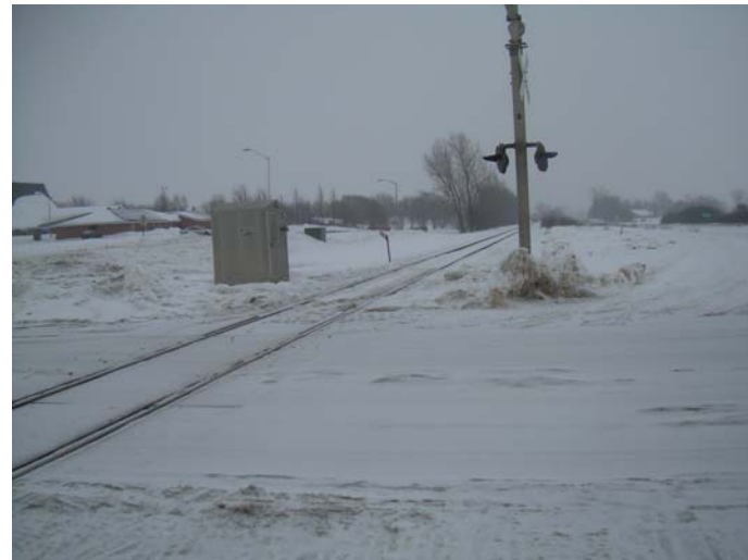
Looking Northeast, Southwest of the Crossing
